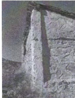
Figure 9. Gypsum pillars in a traditional construction from Rincón de Ademuz (Valencia), 2015. Photo: Vegas & Mileto
