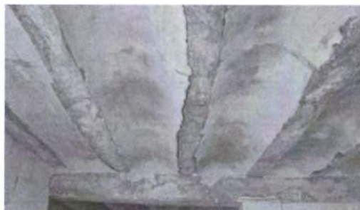
Figure 8. Ceiling with wooden beams filled in with gypsum in a dwelling in Sesga (Rincón de Ademuz, Valencia), 2015. Photo: La Spina
