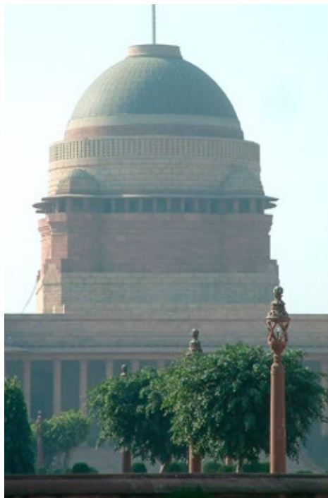
Figure 11. Dome of the Durbar Hall designed by Lutyens in the Viceroy’s House, New Delhi, comprising of three domes one on top of the other: the inside one made of thick brick fabric, the middle one a dome-shaped cone also made of brick and the outer one of reinforced concrete covered with waterproof copper sheets (Vegas 2006).
