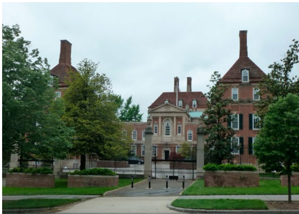
Figure 12. British Embassy at Washington D.C. (1925-1930) designed by E. Lutyens and construction supervised by Frederick H. Brooke (Vegas & Mileto 2013).
