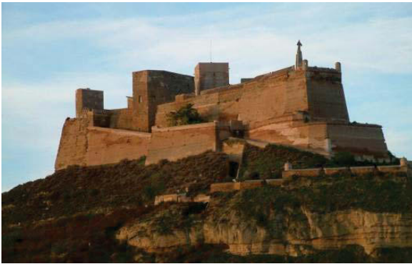
Fig.1 - General view of the castle of Monzón (Huesca) from the north-east
