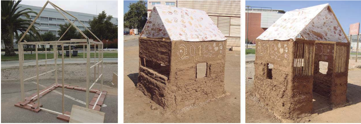
Fig. 1. Start and end of the group construction.
