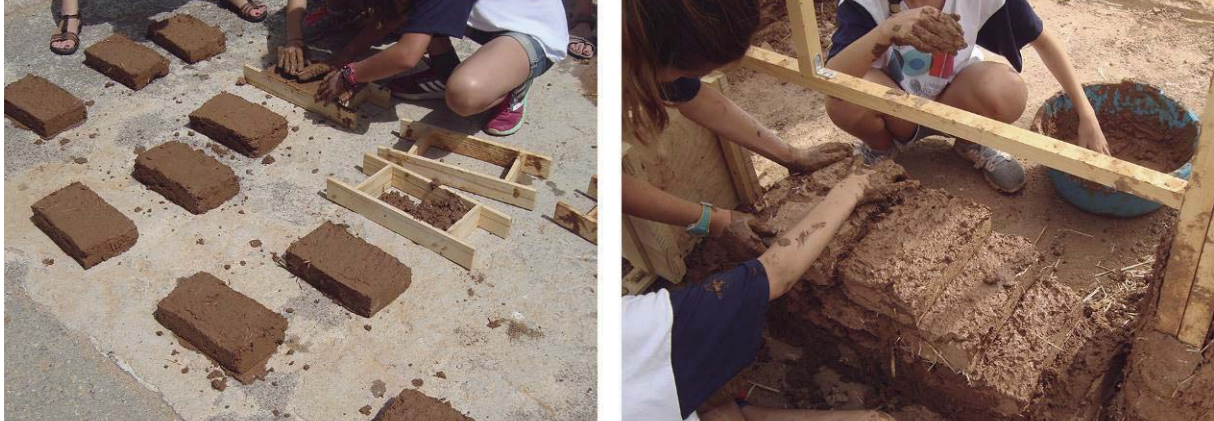
Fig. 6. Adobe production and construction process.
