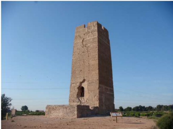
Fig. 20. Bofilla Tower after restoration (C. Mileto and F. Vegas).
