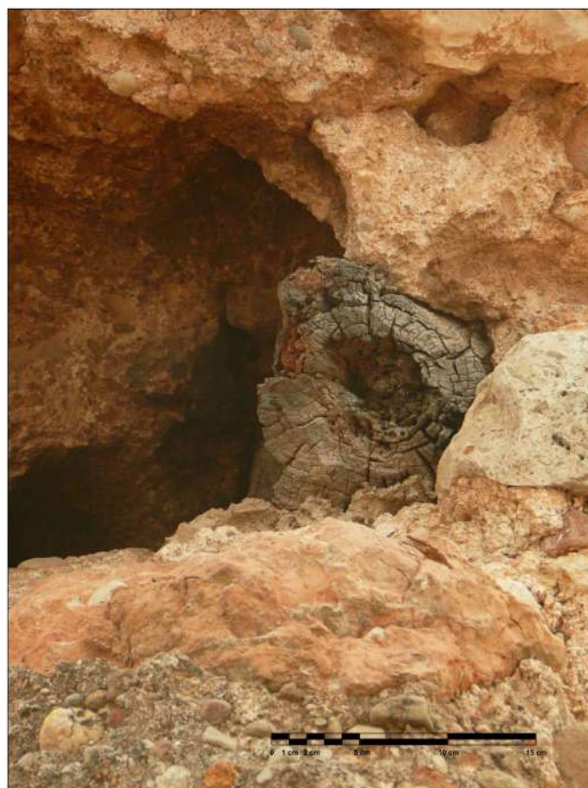
Fig. 5. An example of wooden sleepers in the corner of the northwest wall (V. Cristini).
