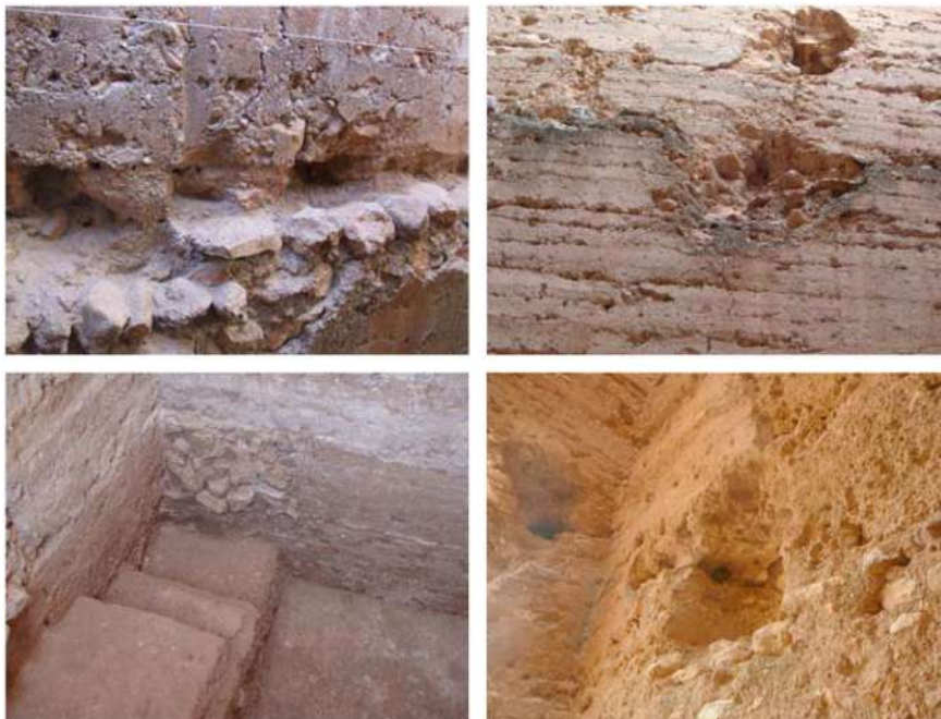
Fig. 7. Study of the imprints that the original floors left on the internal walls of the tower. It has been possible to understand the location of the girders and joists in every floor and the place where the ladders were placed (C. Mileto and F. Vegas).
