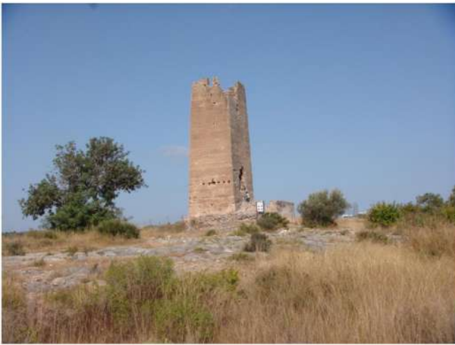
Fig. 1. Bofilla Tower before the conservation work (C. Mileto and F. Vegas).
