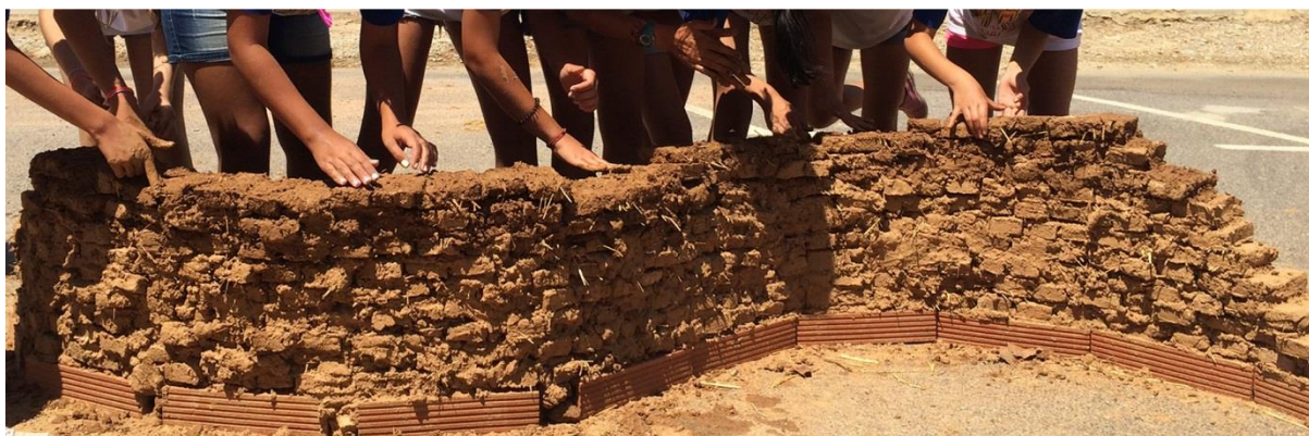
Fig. 6. Image of the wall construction
