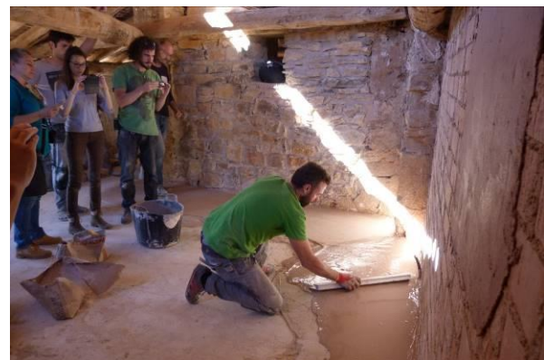
Figures 7 and 8. Students working on their flooring samples and on the gypsum flooring in the room
