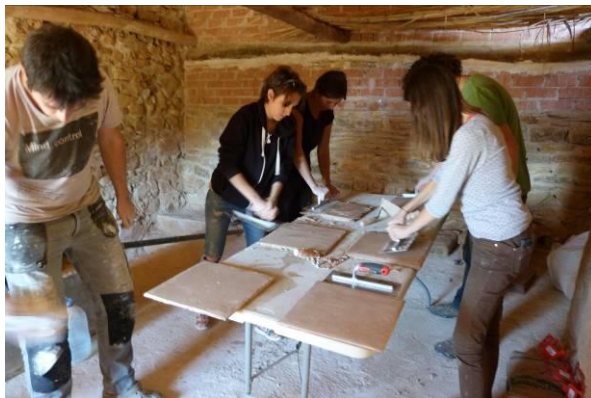
Figures 7 and 8. Students working on their flooring samples and on the gypsum flooring in the room
