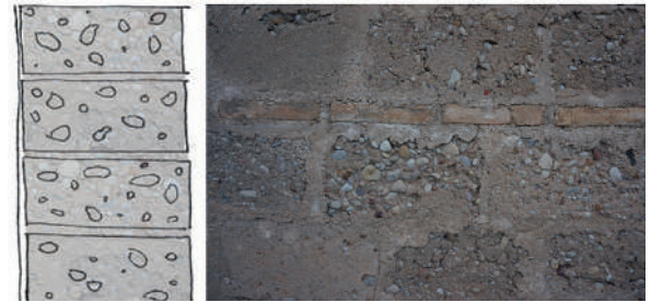
Fig. 7 Detail of a wall of binder-earth blocks
