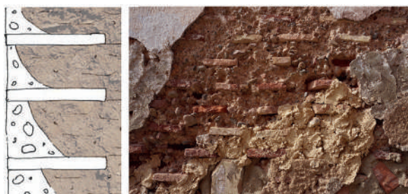
Fig. 4 Detail of a type II Valencian rammed earth walls
