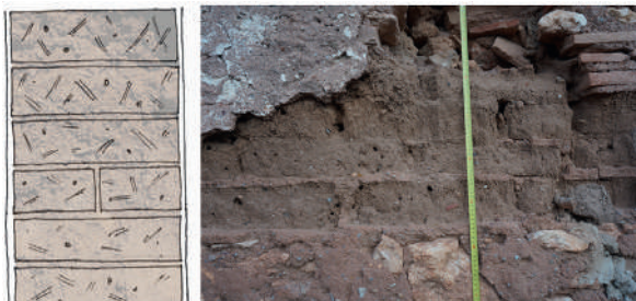
Fig. 6 Detail of an adobe wall
