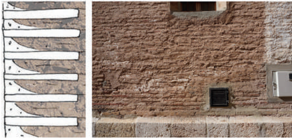
Fig. 5 Detail of type III Valencian rammed earth wall
