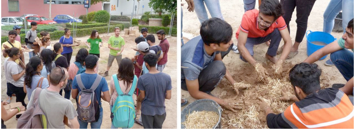
Figure 1. Left: Image of students at the start of a practical workshop. Right: Preparation of adobe mix.
