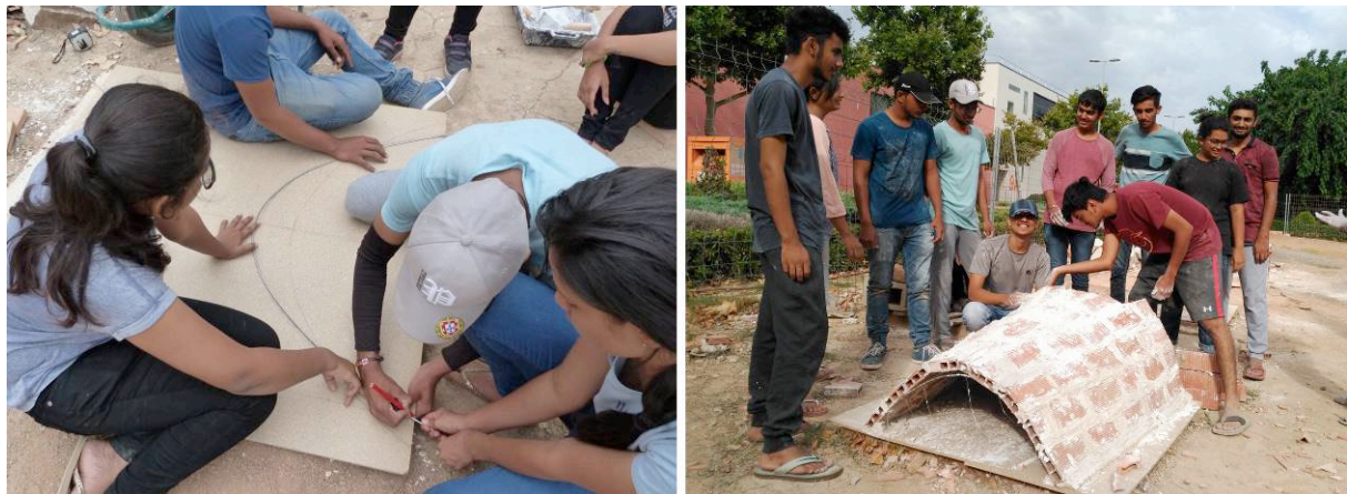
Figure 3. Left: Workshop on the design and outline of tile vaults. Right: Vault construction workshop
