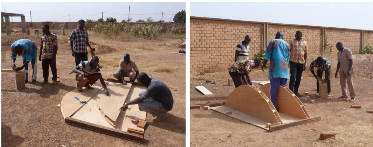
Figure 1. Placement of wooden centring.
