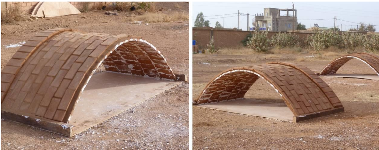
Figure 3. Final result of the vaults.
