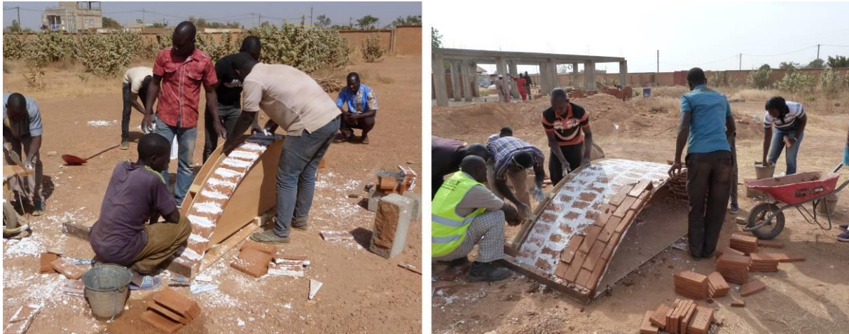
Figure 2. Construction of vaults with CEBs.
