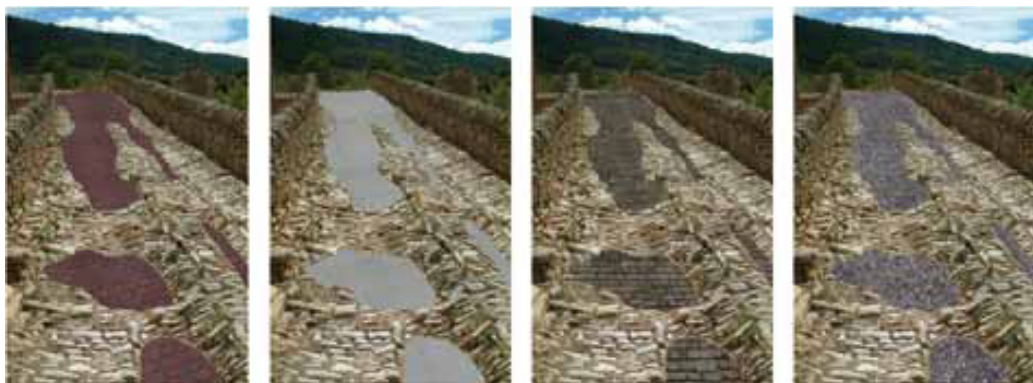
Fig. 5 Medieval bridge in Poble de Ballestar in Castellón (Spain). Several computer options done to test the impact of different ways of filling in the gaps in the pavement.
